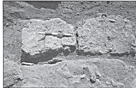
3. The bedding of the central aisle disconnected by 20 centimeters horizontally.
